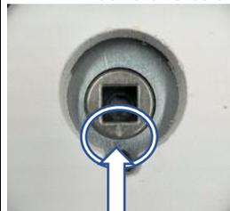
Ensure this arrow is pointing down when installing exterior housing
